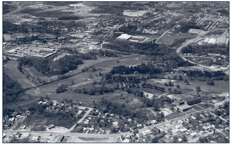
Gillespie Golf Course anchors this 1956 image of southeast Greensboro, an area that has recently experienced both renovations and new construction.
