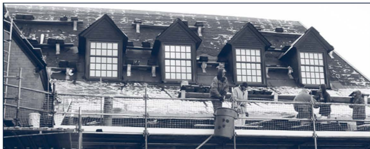
Contractors work despite freezing temperatures and snow, November 2008
