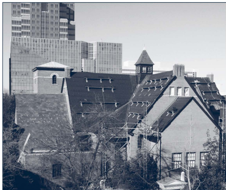
Parts of 1892 roof facing cemetery prepared for reinstallation of slate, January 2009
